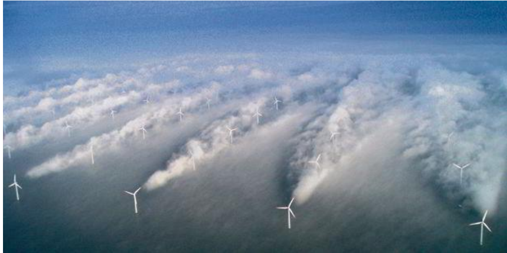
Fig. 2: A picture to show the wake interferences among wind turbines in an offshore wind farm.
